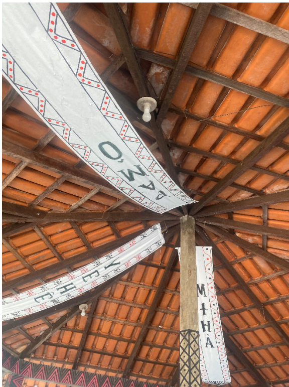
Figure 5 The roof of the Amarn community
