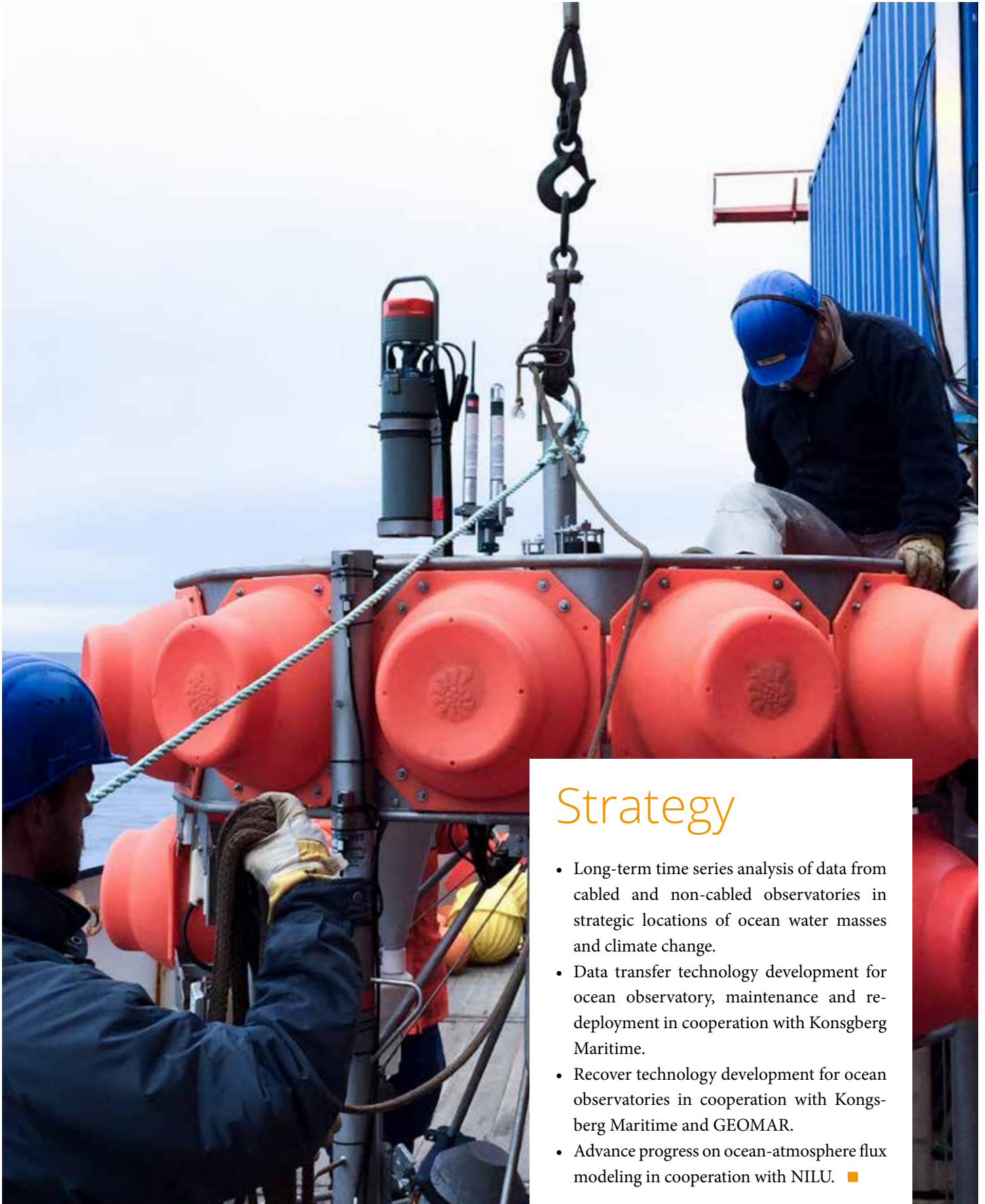
Deployment of CAGE methane sensor from the RV Polarstern to the Hausgarten deep-sea observatory in the Fram Strait. The deployment was conducted within the EU project FixO3 in which CAGE participates. Photo: Kasia Zamelczyk.
