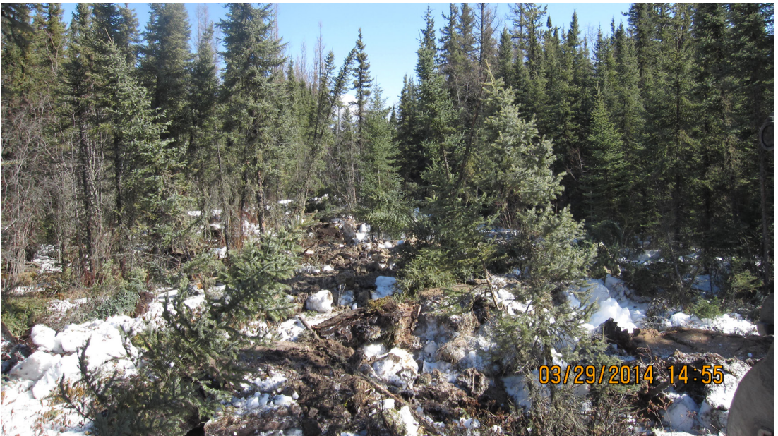
Figure 6. Lease road after treatment with mounding, tree-felling, tree-bending, and tree transplanting. Photo courtesy of MEG Energy.
